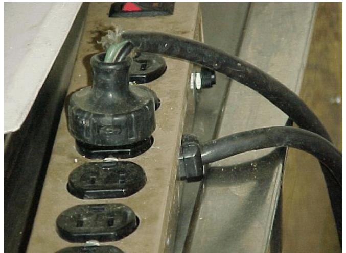
*The power cord above has had its protective sheathing torn away from the plug head, exposing energized wires.*
